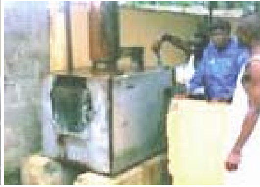
Dismantling of the heat chamber at Rukpokwu
