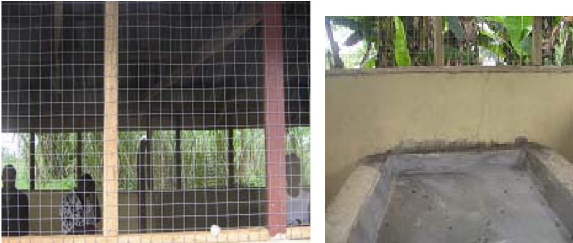
Figure 2: Galvanized wire mesh installed and fryer orientation corrected at Otor- Iyede
