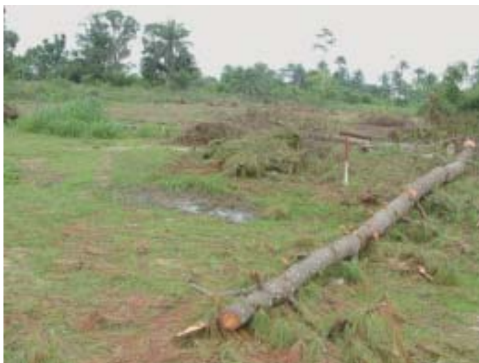
Cleared site for CMD postharvest model plant at IITA Onne.
